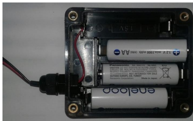
Photo 9 – Replacing battery in battery box
